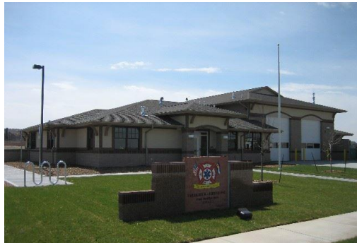
Station 3 6800 Tilbury Avenue Firestone, CO 80504
